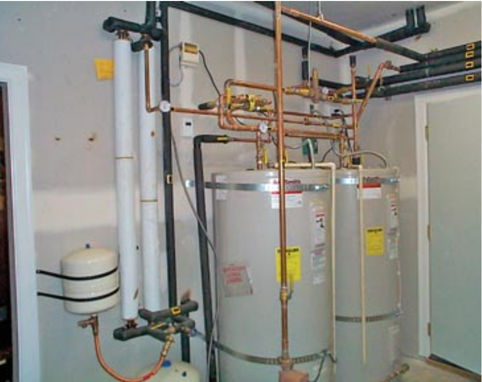
Two 120 gal. storage tanks showing solar heat exchanger and injection loop for Warmboard heating system
