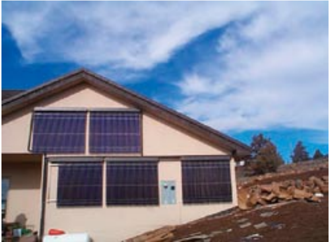
Millers’ 150 tube THERMOMAX solar heating system. They are mounted vertically on south wall to help eliminate summer over- heating
