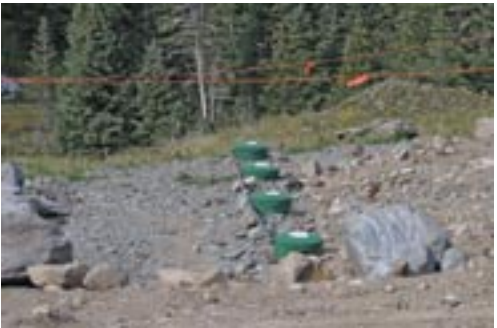
Buried in the bedrock are four one thousand gallon propane tanks
