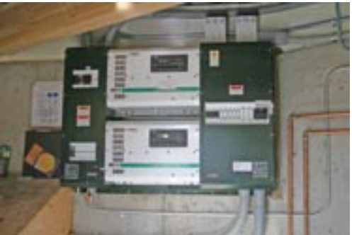
Two Xantrex 4024, (Center) Outback DC (left) and AC (right)
