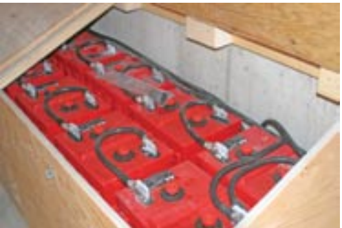
12 Rolls Surrette 4ks25ps Series 5000 Batteries
