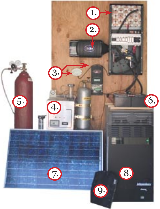
1. Maxwell PC2500 Boostcaps enclosed in a Outback PSDC 2.Outback FX2024 Inverter. 3. Outback Mate and MX60 Controller 4. PEM Electrolizer 5. Hydrogen K tank. 6. Four Hawker Batteries 7. Photovoltaic panel 8. Avista Independence 1000w fuel cell. 9. Plug-in fuel cell stack.
