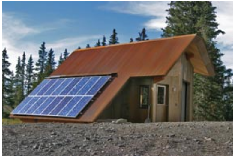
The powerhouse. The heart of the Burr residence energy station. Shown are the 16 BP 150 watt solar electric panels.
