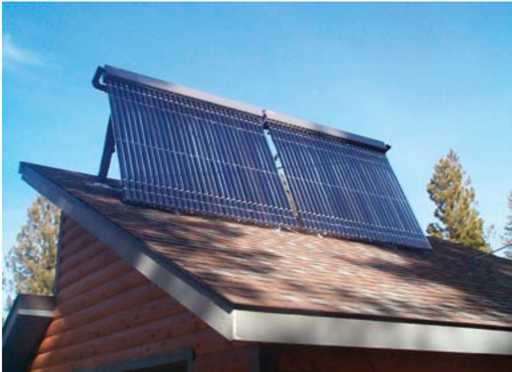
Two 30 tube THERMOMAX evacuated tubes with manifolds
