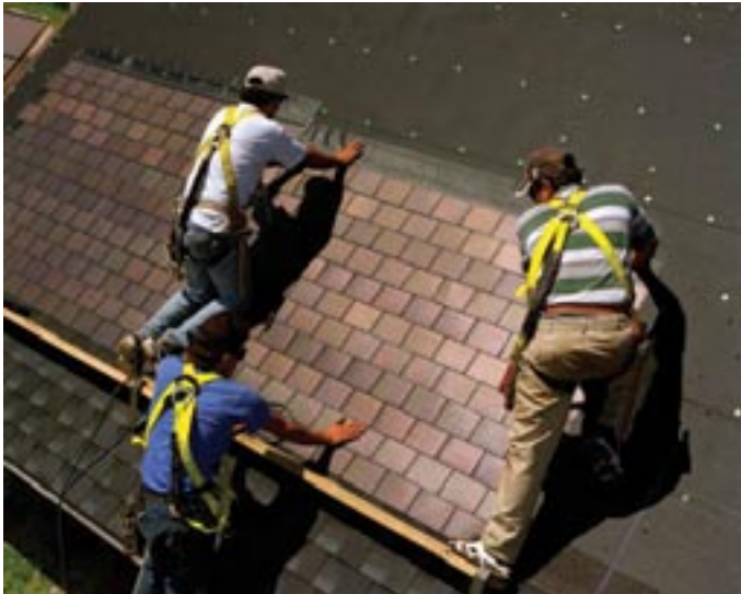
PV professionals install the latest in Photovoltaic roof shingles
