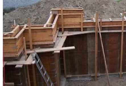
**16. Strip Foundation:** Usually the day after the concrete has been poured the foundation can be stripped. The Concrete company should be called to pick up their forms.
