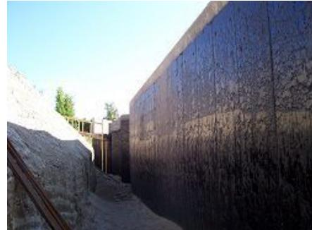
**17. Damp Proofing:** Water proofing is required on the part of the foundation where the slab or skim coat is below grade level.
